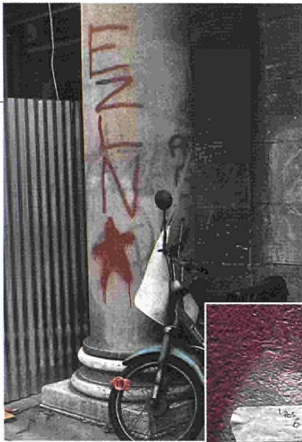
Rome - Cleaning up graffiti : state of damage and parameter determination test.
