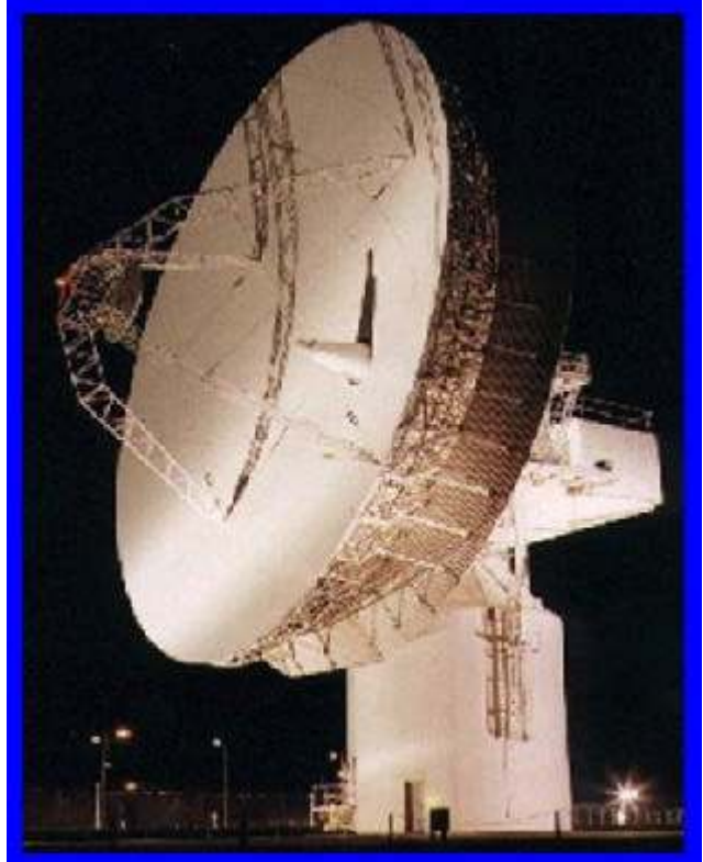
GCHQ constructed an identical "shadow" station in 1972 to intercept Intelsat messages for UKUSA
