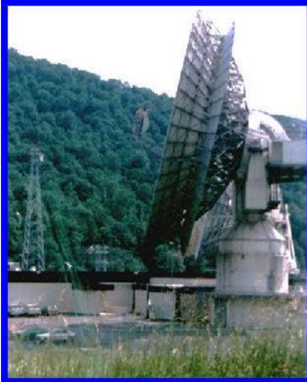
Satellite ground terminal at Etam, West Virginia, connecting Europe and the US via Intelsat IV
