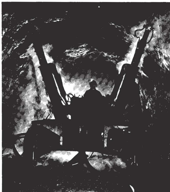
A modern drilling machine makes two blasting holes at a time in an LKAB iron ore mine, Kiruna, Sweden. Behind Danish and Norwegian arguments against a Nordek common external tariff, "lies the fear...that Swedish industry, often more advanced and stronger financially and technologically, might stage massive take-overs of companies in the other countries." ©LKAB Fotograff. Courtesy of the Swedish Information Service, New York, N.Y.
