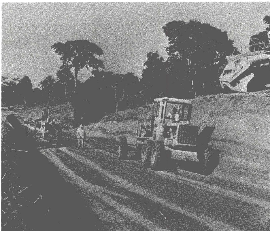
Landmovers level the ground on which tracks will be laid for the Cameroon rail extensions.
