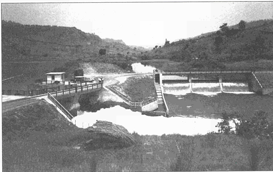
The dam and (left) the flow regulator were separated to facilitate the diversion of the Ruzizi waters during the construction phase
