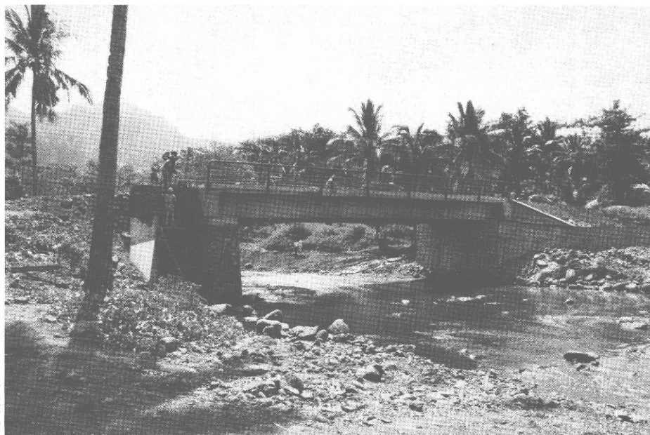
Finishing stages in the building of a new bridge at Pomoni; the old bridge had been destroyed by rocks and mud coming down the mountain following torrential rains
