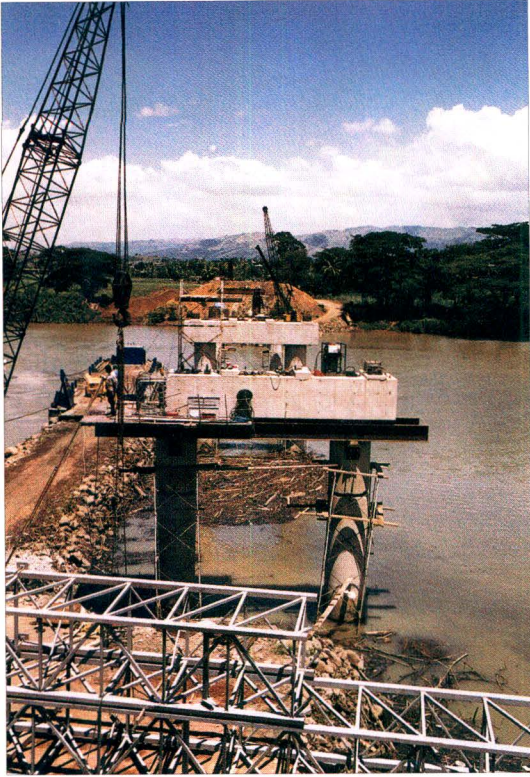
Ba bridge under construction
