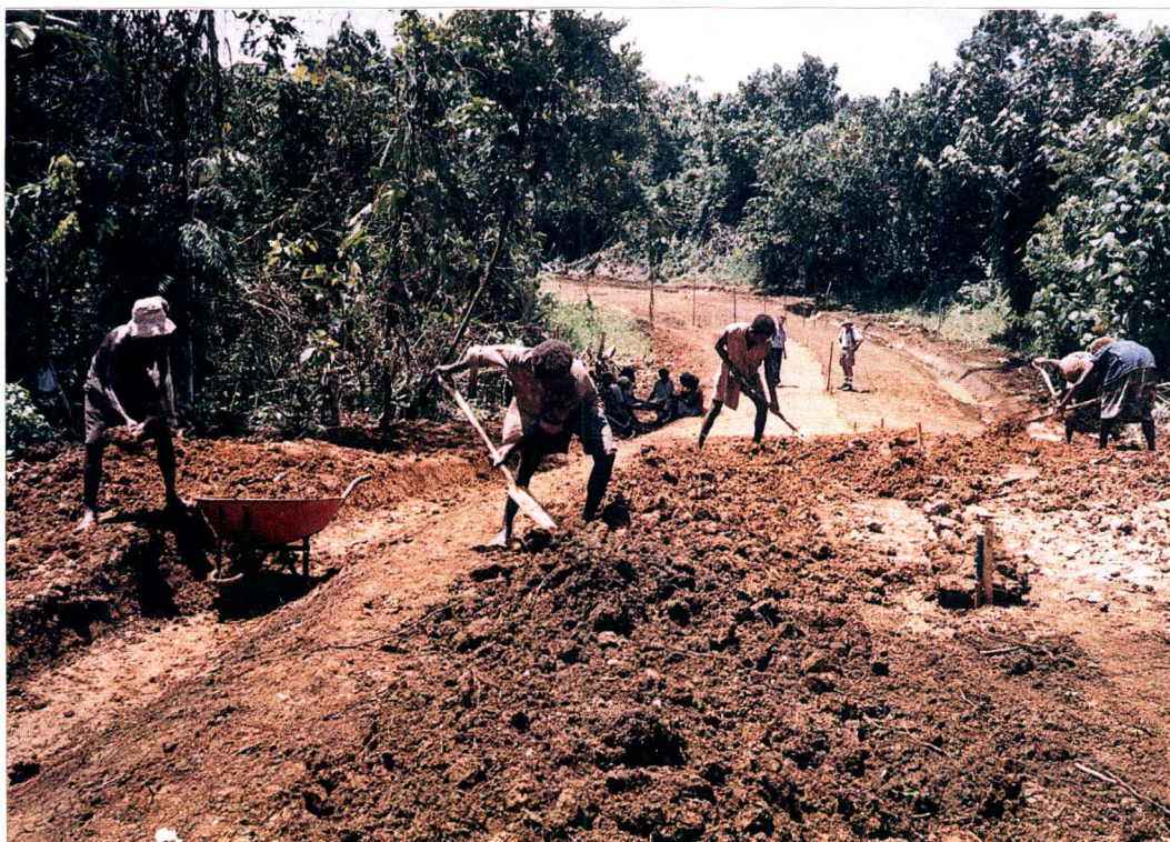
Road construction by manual labour
