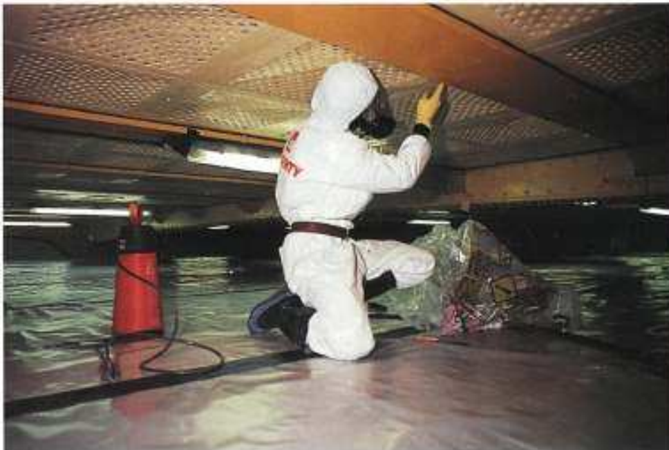
The Directive seeks to encourage the removal of asbestos from buildings.
