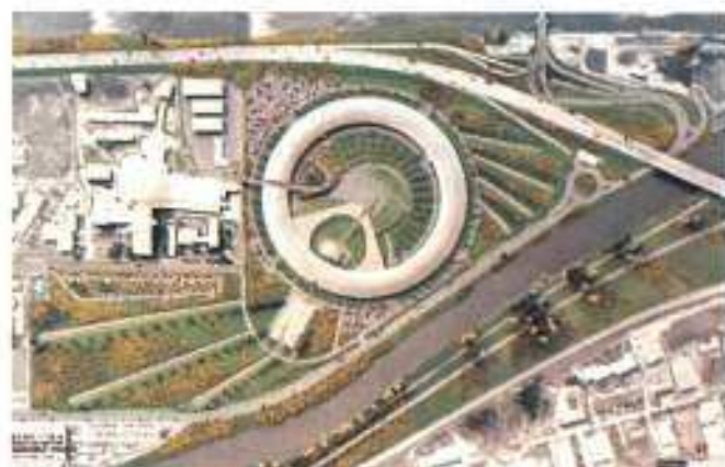
Building the Synchrotron at Grenoble: a pilot site for the prevention of accidents at work.
