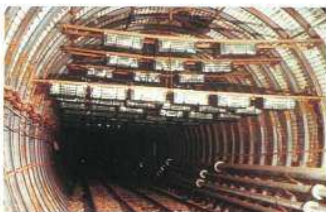
Water-trough explosion barrier: a safe means of suppressing explosions and limiting their spread.
