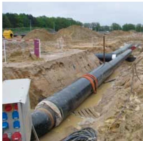
Trench and pipeline construction
