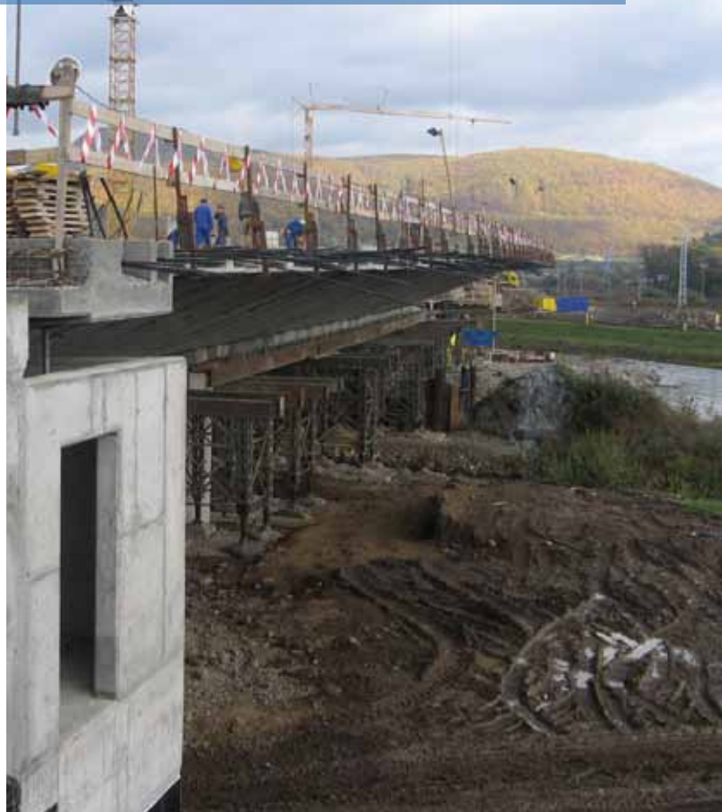
Žarnovica-Šašoske-Podhradie R1 expressway, Slovakia
