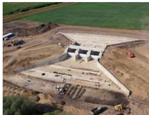
Example of two water reservoir inlet structures
