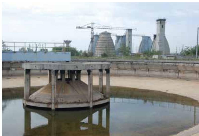
Bucharest wastewater infrastructure, Romania
