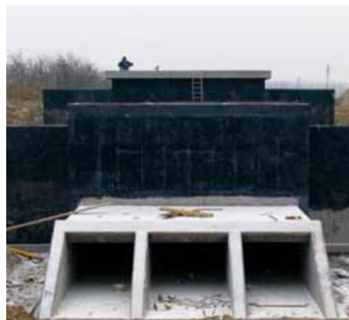
Flood reservoir dyke to be constructed
