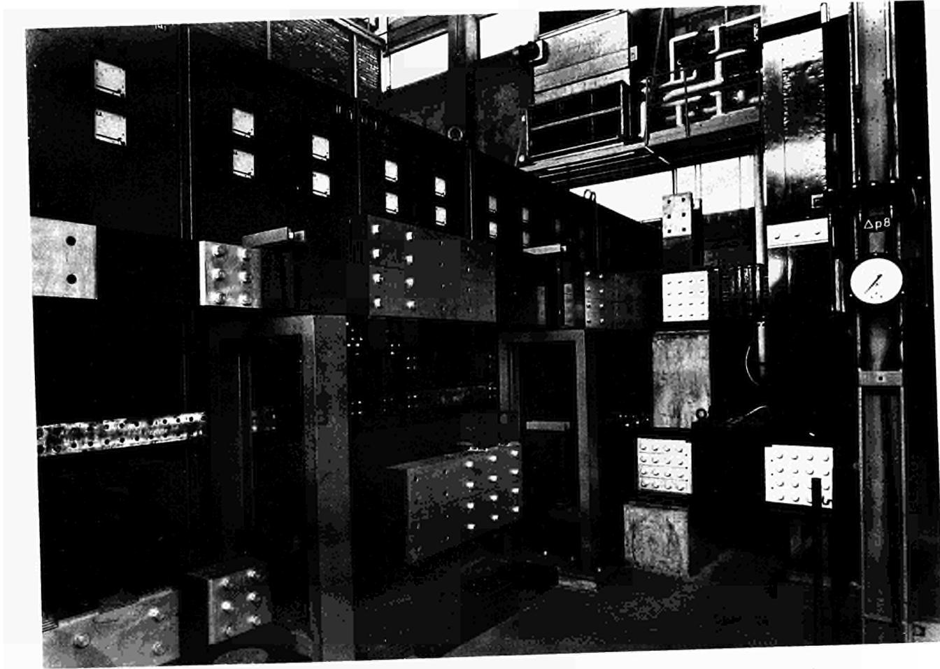
Fig. 5 Rectifier group with current bars and Iso-shunts
