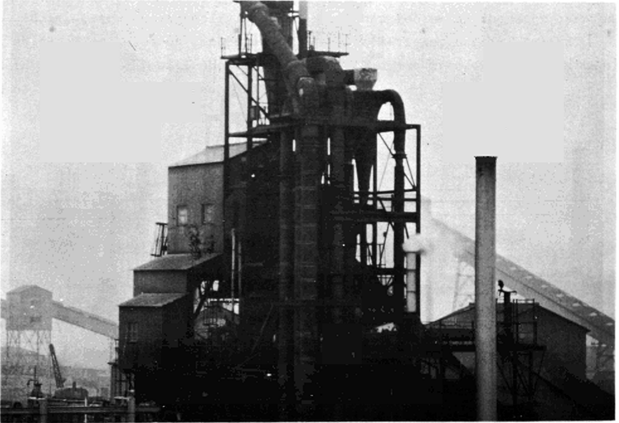
Figure 3 - 10-Tons oven during charging the preheated coal
