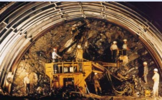
Building the Athens metro
