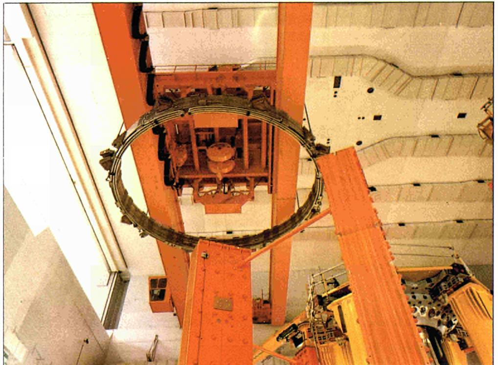
*The 150 tonne crane transferring one of the largest outer poloidal field coils to the Torus Hall*
