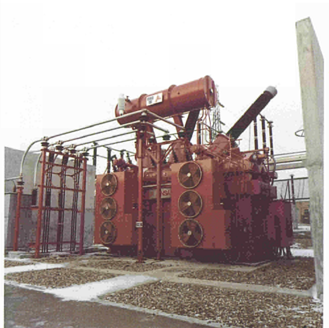
Fig. 17 The 400kV/33kV substation showing the third arrestor-transformer system installed.
