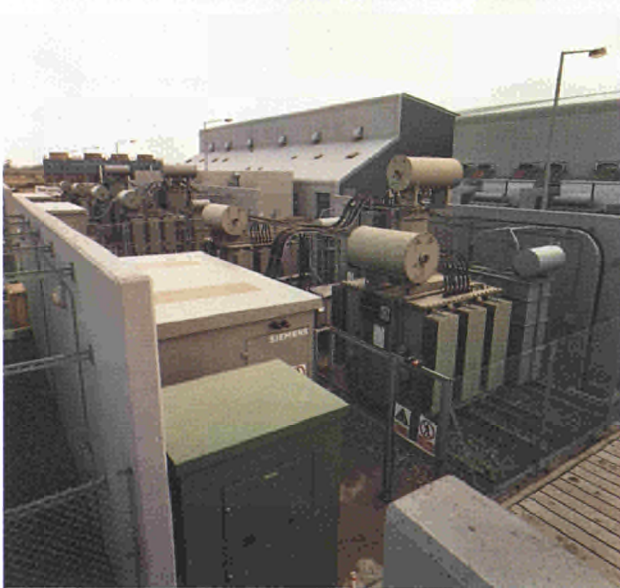
Fig. 12 The outdoor high voltage grid power supply modules for JET's neutral injection system.
