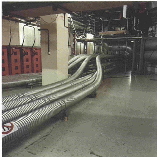
Fig. 14 The SF 6 transmission lines in the Torus Hall Basement.
