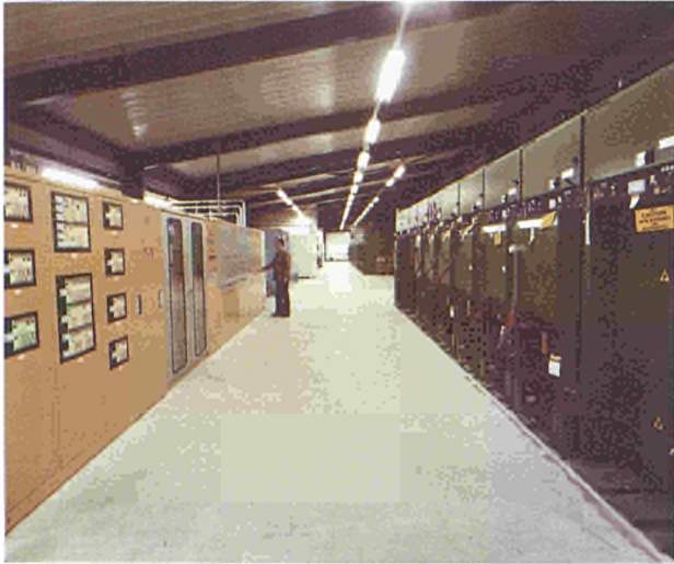
Fig. 18 The extension of the 33kV switching system, showing the new 33kV, SF_6 Breakers.
