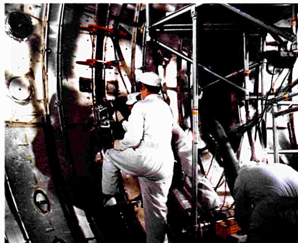
Fig.6 Welding of the torus U-joints, the vacuum seals, between octants.
