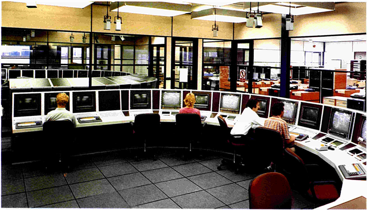
Fig. 27 Machine subsystems consoles in machine control room.
