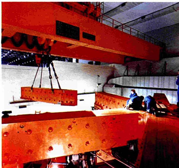
Fig.5 The final upper horizontal limb being installed in January 1983 to complete the magnetic circuit.
