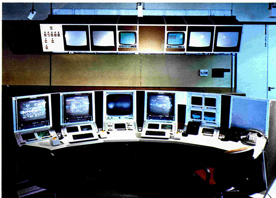
Fig.26 JET machine control room console with synoptic viewer above.
