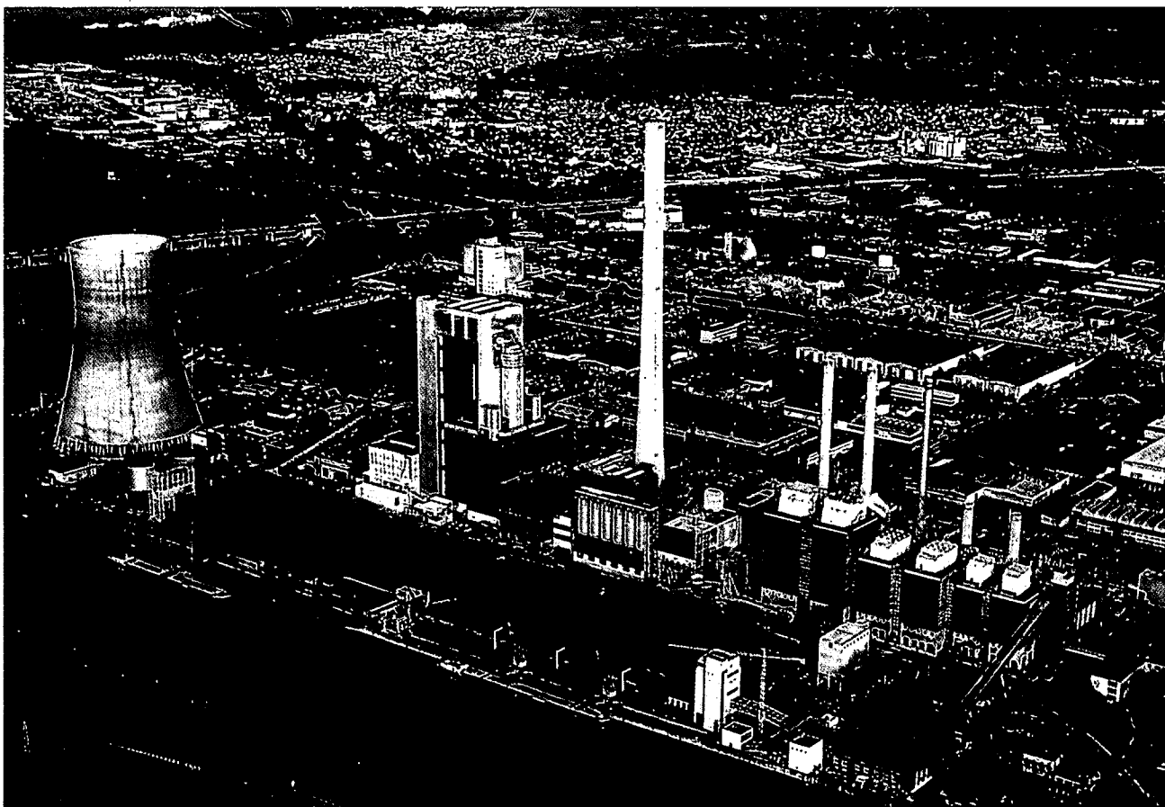
EVS power station at Heilbronn
