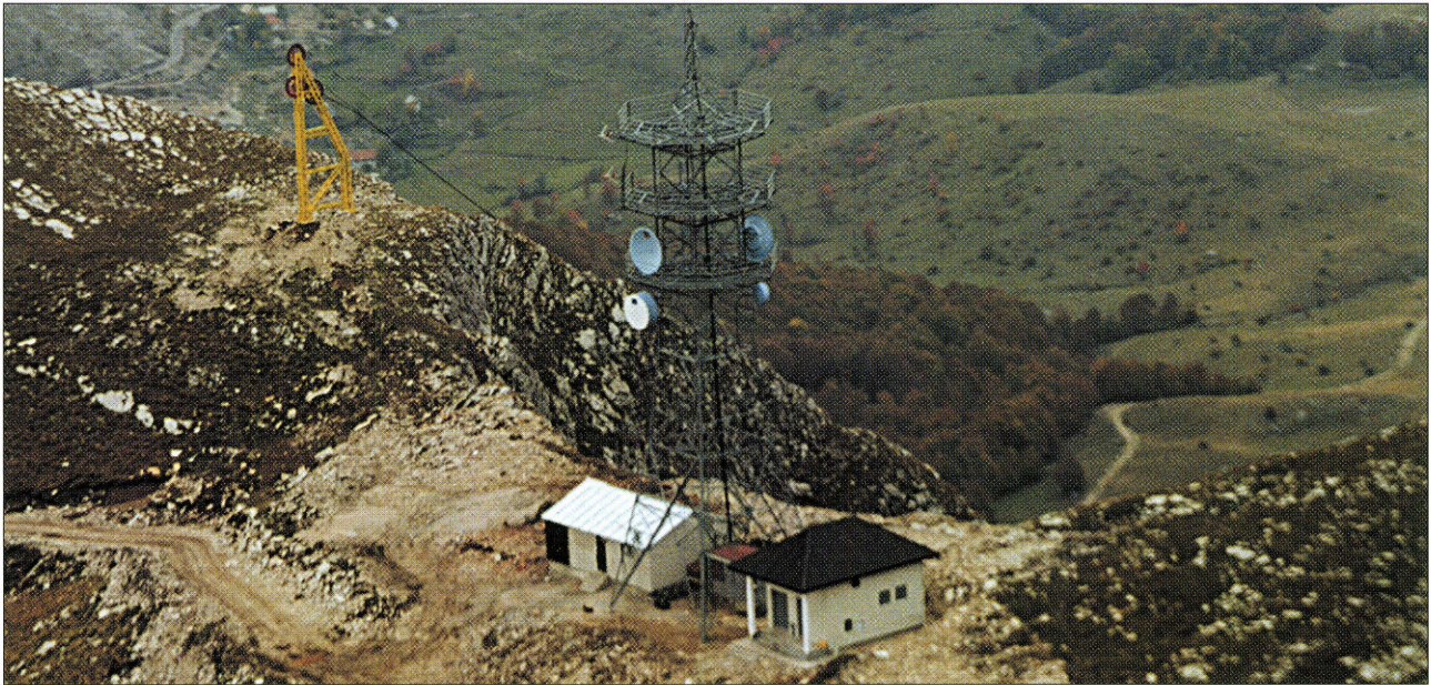
Not all 32 radio-relay links put in place by the EU programme are quite so remote
