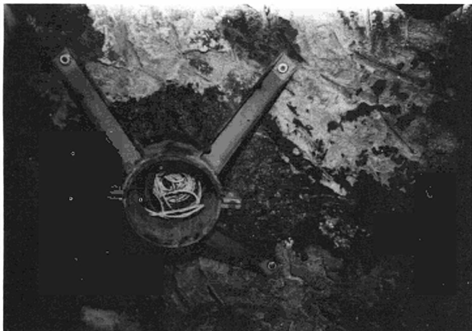
Fig. 28 : Oil ducts of a pressure cell and sleeve before concreting
