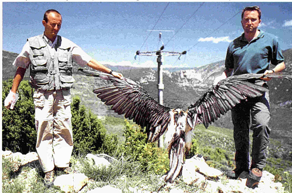
Electric powerlines responsible for electrocuting bearded vultures. Photo: F. Marquez
