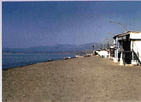
Illegal summer houses along a beach in Lakonikos bay. Photo: STPS
