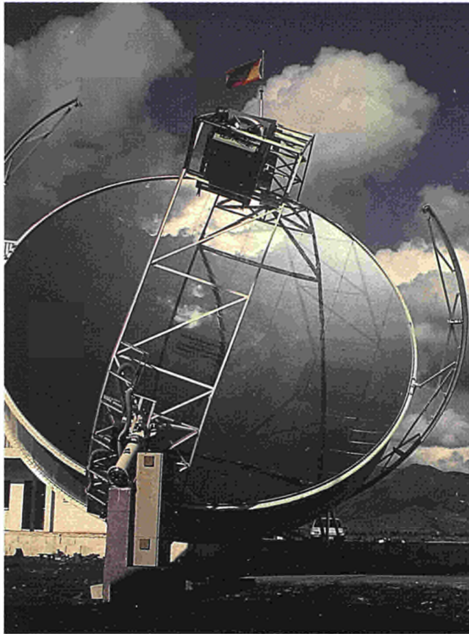
Parabolic mirrors concentrate the sun's rays in the centre of the dish
