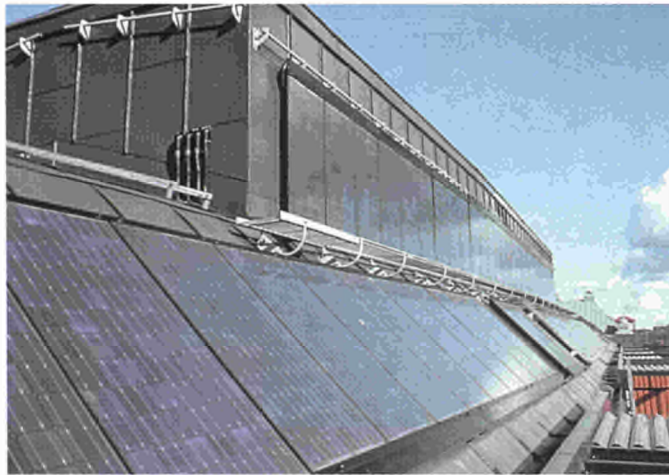
A PV power plant in Sweden
