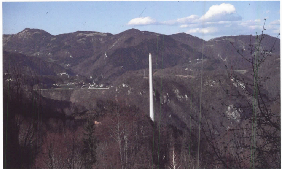
To disperse emissions from the Trbovlje power station in the Sava Valley, a 362-m chimney was built in the 1970s (Photograph: Karel Natek)
