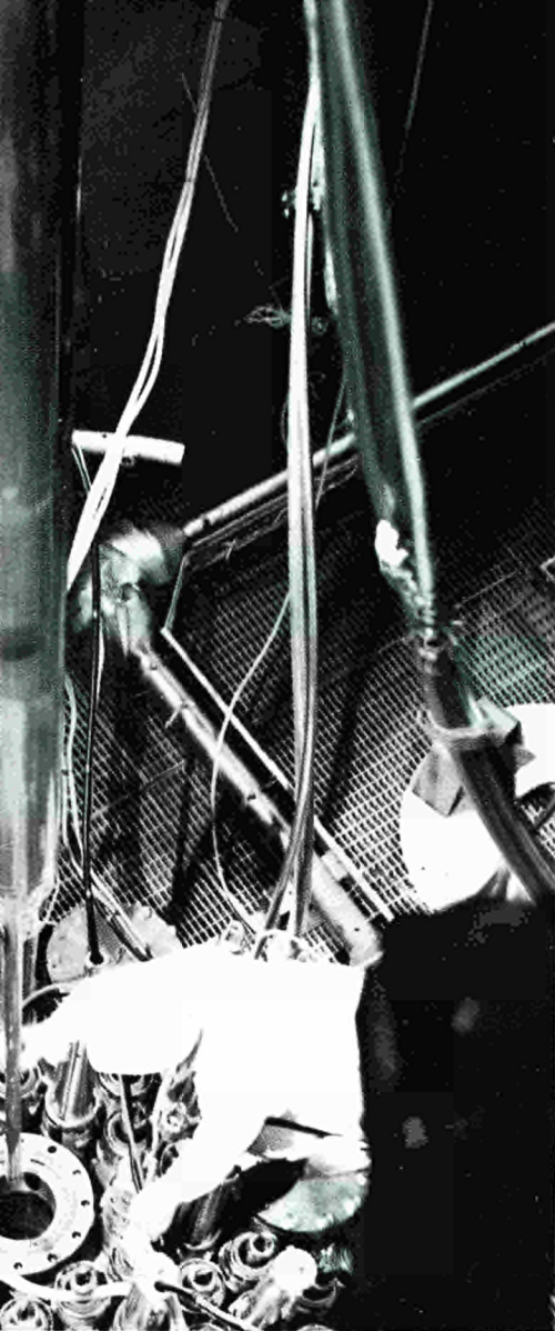
Introduction of a sodium loop into the central channel of the BR-2 reactor
