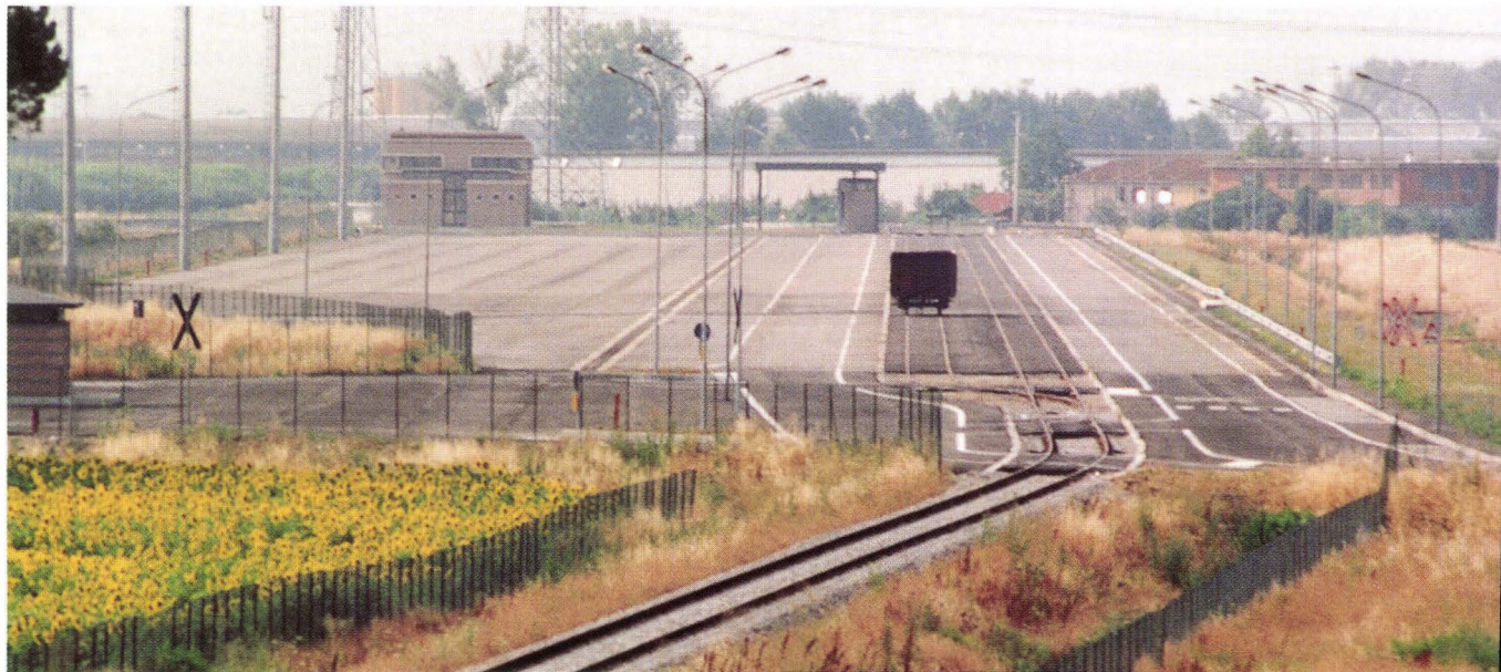
Transfer from train to lorry in a flash
