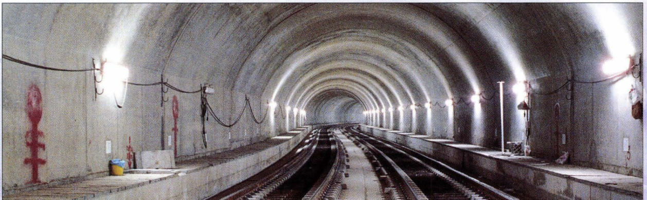
The underground takes shape bit by bit
