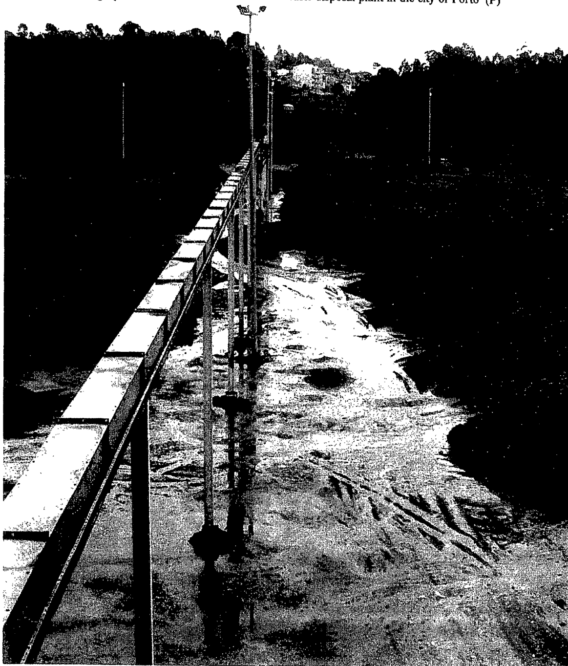
Photograph N°5 Construction of the 2nd waste-disposal plant in the city of Porto (P)
