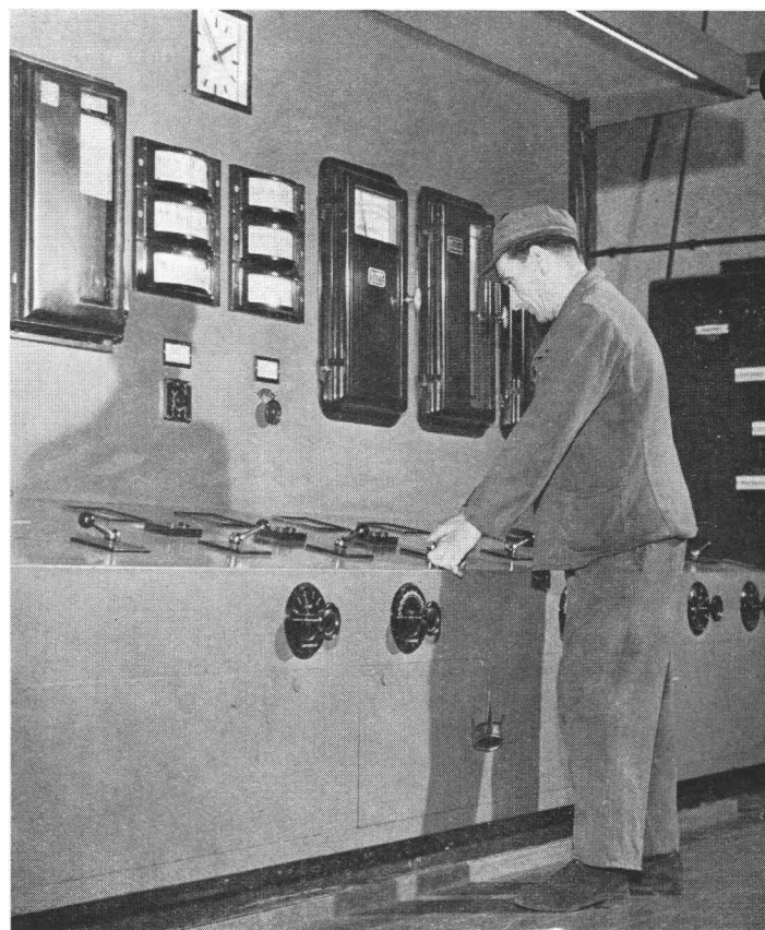
The automatic control panel of an Askania boiler at the Dortmund-Hoeder Huetteneverein, Germany. The more efficient use of fuel is one of the aims of the technical research programme.
