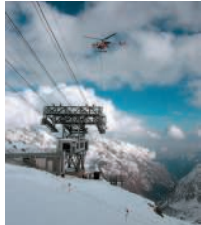
Monitoring avalanches in Alagna (Italy)
