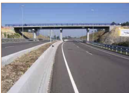
The first European fully vehicular highway carbon fibre composite bridge was installed in Spain
