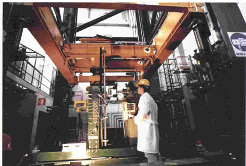
Fig. 6.2 The facility ROBERTINO.
