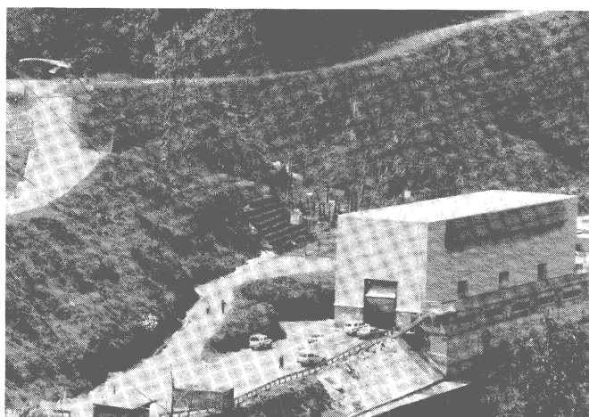
Monasavu Hydro-Electric Scheme—Wailoa power station.
