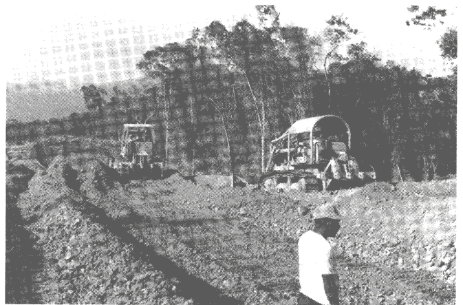
Hiritano Highway under construction.
