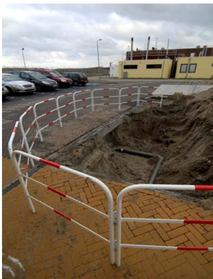
Example of excavation work at JRC-IE for which a work permit is required.
