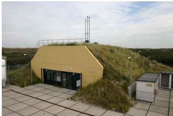
The High-Pressure Tank Testing Facility integrated into the landscape
