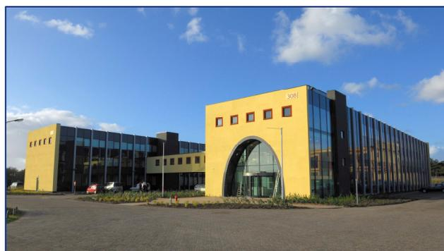
aluminium curtain walls of enhanced thermally insulating glass with a heat reflecting coating and a good solar and daylight penetration factor. Special attention was paid to obtain a harmonised picture following a specific colour scheme and emphasizing the arched entrance as new focal point. A new passageway connects the two twin buildings.
