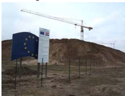
Construction site entrance
