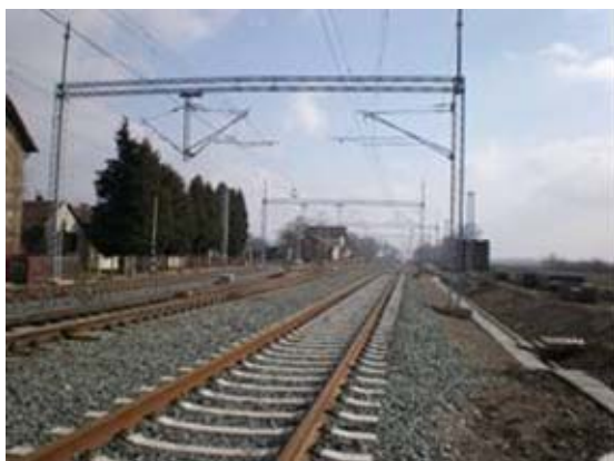
Section of reconstructed railway
