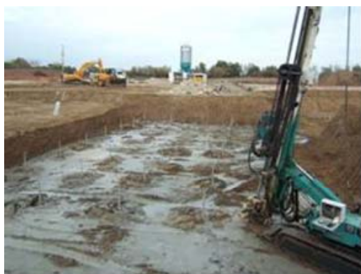
Excavation and piling works
