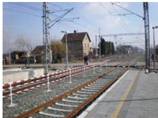
Deletovci Station looking East
