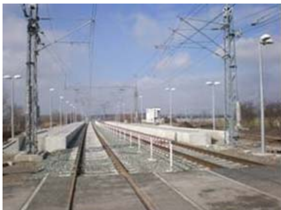
Deletovci Station looking West
