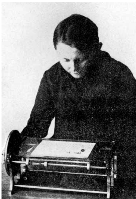
Optometer to test eyesight and ability to judge distance.
