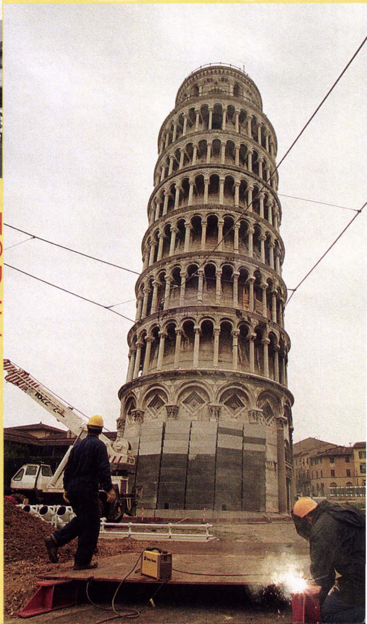
(Top) The famous Leaning Tower of Pisa circa 1958. (Bottom) In January 1999, workers prepared to remove soil from under the tower.
