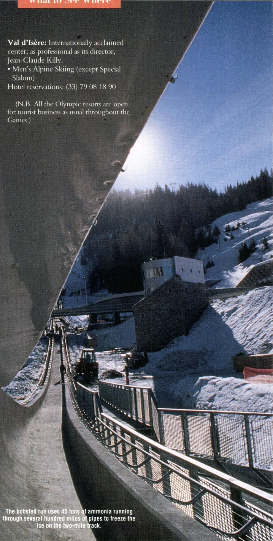
The bobsled run uses 45 tons of ammonia running through several hundred miles of pipes to freeze the ice on the two-mile track.
