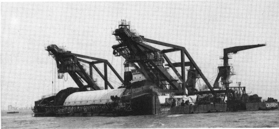
barrier is now being built, at a cost of approximately \$1.5 billion. The design—which is unique, according to Dutch engineers—calls for sliding gates in the three tidal inlets. This will enable the Oosterschelde to be closed in bad weather, while letting the sea water flow in and out during normal conditions, thus preserving tidal movements, the environment, and fisheries.
