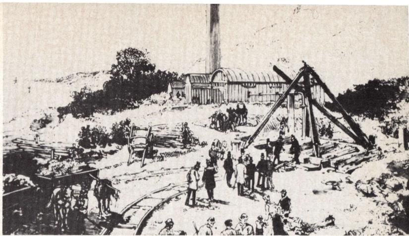
*Sinking an operational shaft for Chunnel construction at St. Margaret's Bay on the Kent Coast in the 1870s.*
