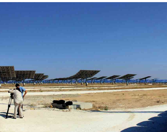
THERMOSOLAR GEMASOLAR Construction of small-scale concentrated solar power plant (17 MWe) in La Monclova between Córdoba and Seville, Spain
