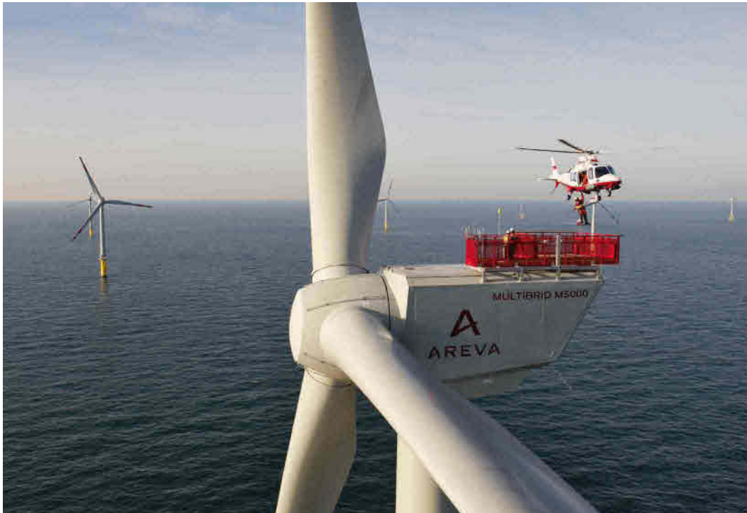
GLOBAL TECH | OFFSHORE WINDPARK Construction of 400 MW wind farm north-west of German island of Borkum in the North Sea, Germany
