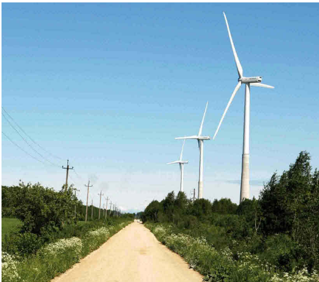
EESTI ENERGIJA GENERATION ENHANCEMENT Construction of wind farms in Aulepa and Narva, Estonia
