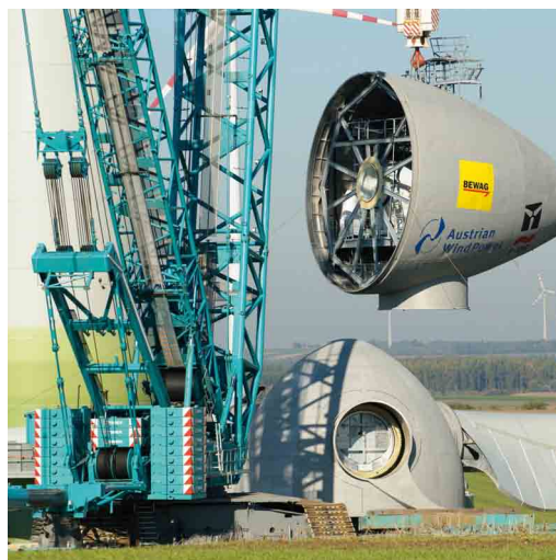
BEWAG AUSTRIAN WINDPOWER Construction of wind turbines in Burgenland, Austria
