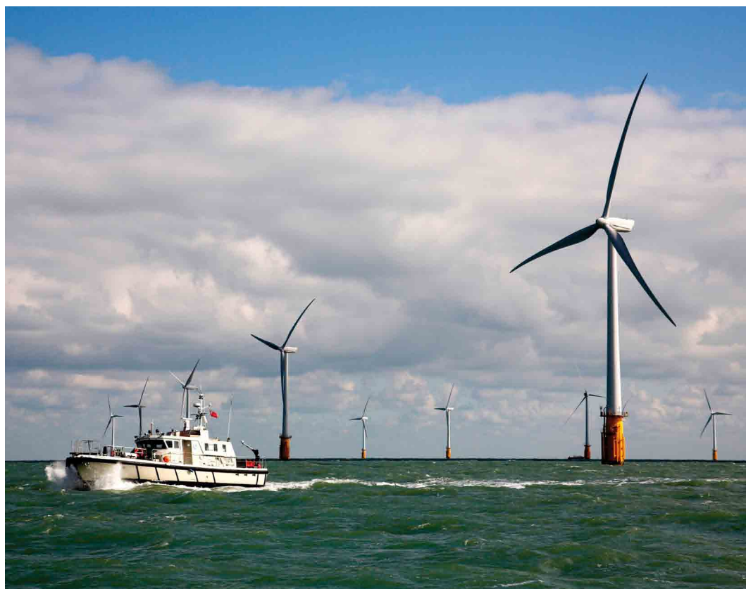
THANET OFFSHORE WINDFARM Construction of large offshore wind farm (300 MW) east of London in Thames estuary, United Kingdom
