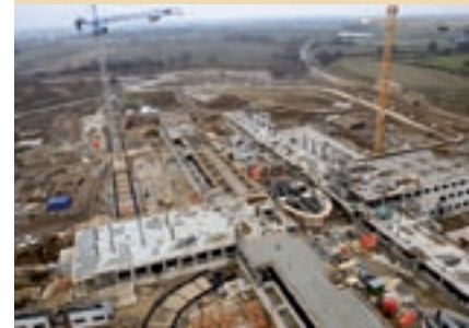
Construction of hospital complex, Sittard
