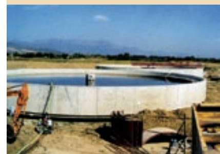
Construction of wastewater treatment plant, Turkey
