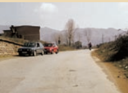
Upgrading of roads, Albania
