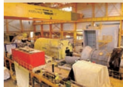
Combined-cycle power plant turbine, Carregado
