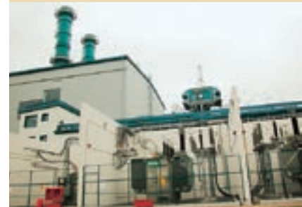
Power plant, Riga
