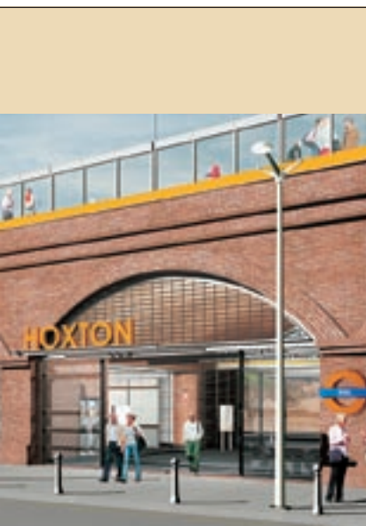
New station on East London line, Hoxton
