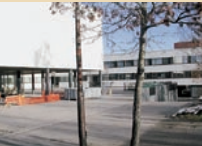
School refurbishment, Oulu region
