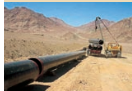
Construction of natural gas pipelines, Egypt
