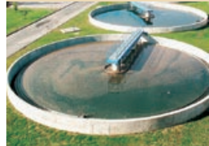
Wastewater treatment, Castilla-La Mancha
