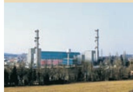
Power plant, Gissi
