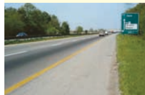
Modernisation of road network in Serbia and Croatia
