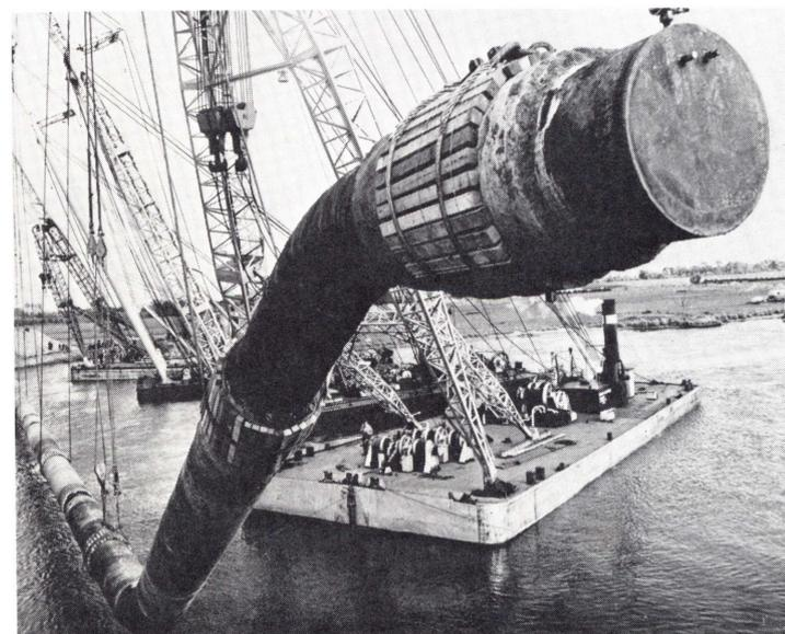
*Floating cranes lay natural gas line under the Yssel River, the Netherlands.*
