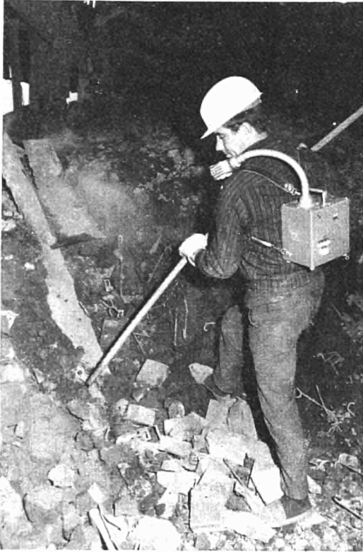
a. In use during the demolition of an open hearth furnace
