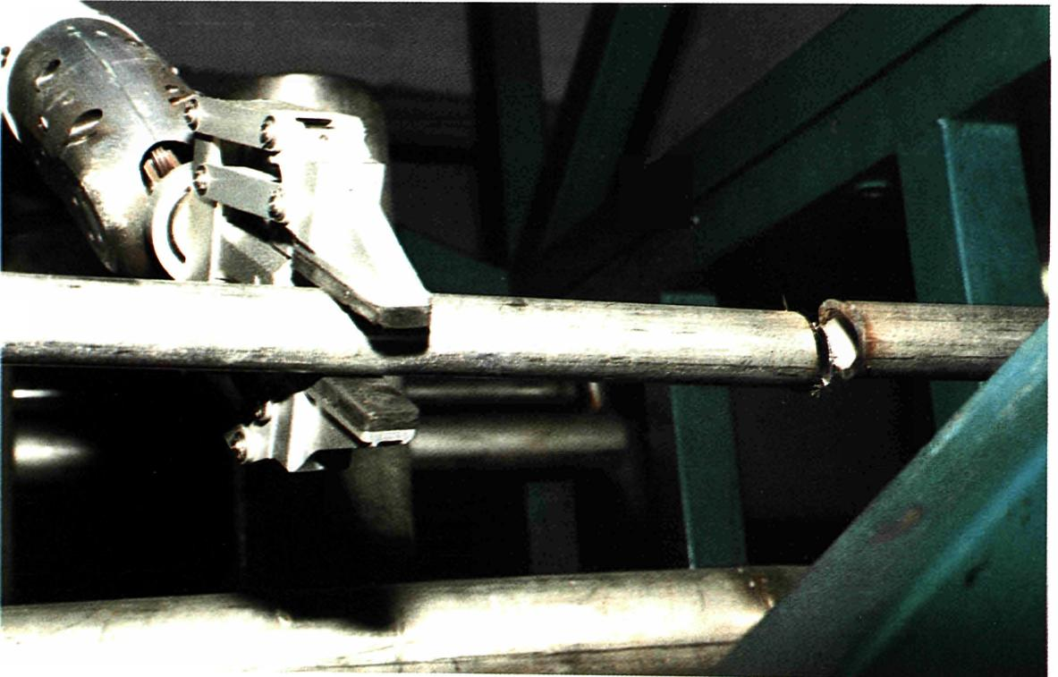
Figure 4 - The cutting of the small piping
