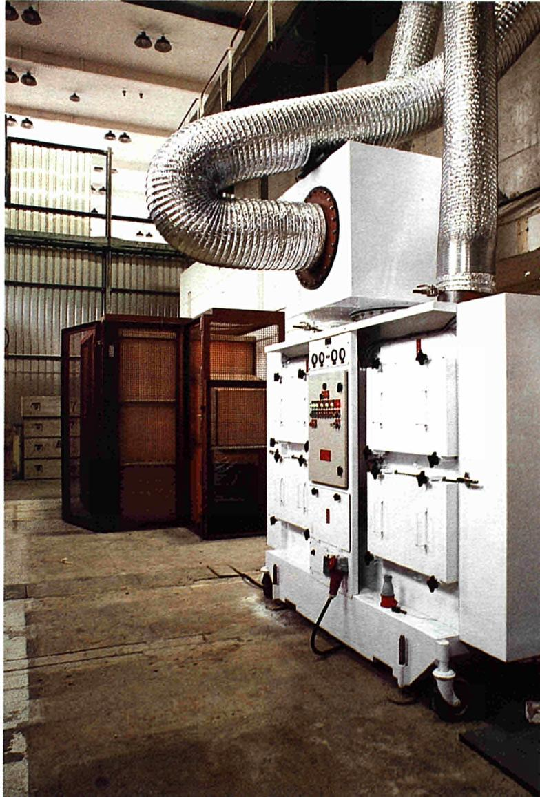
**FIGURE 1 - MOBILE FILTRATION UNIT WITH MAN-ENTRY TO BIOSHIELD
