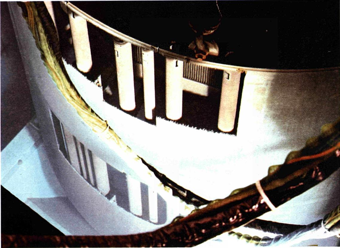
Figure 4: Dismantling of the steam dryer shell by underwater plasma arc cutting
