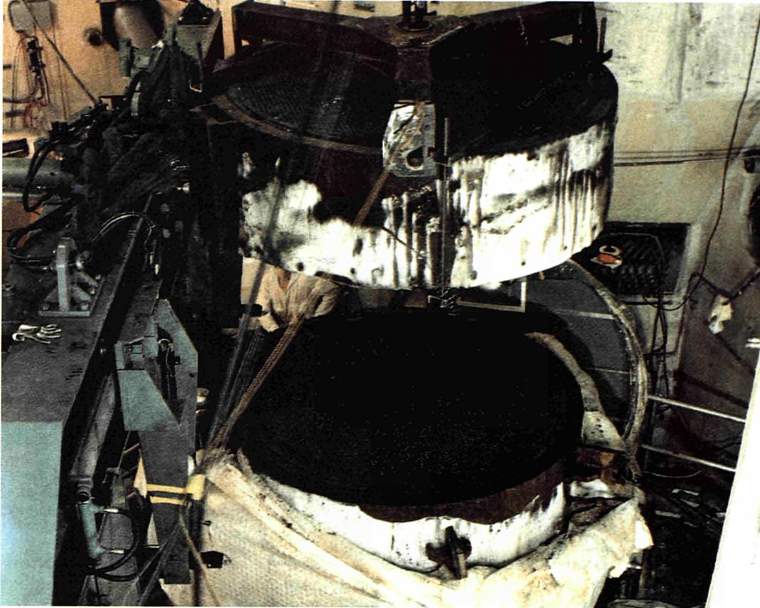
Figure 2: Lifting of an ice-sawed segment of the secondary steam generator
