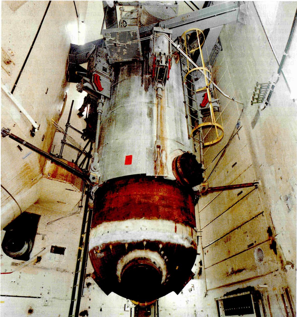
Figure 1: Looproom-2 with SSG-2 after removal of all pipings
