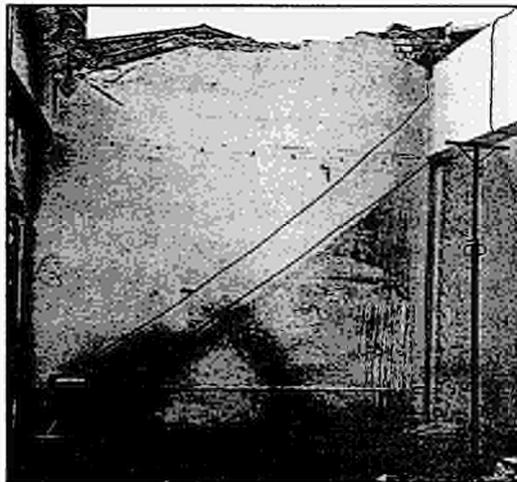
Figure 1: Cutting of a concrete structure with a diamond cable.
