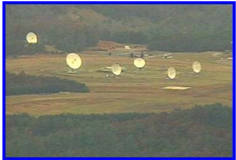
ECHELON satellite interception site at Sugar Grove, West Virginia, showing 6 antenna targeted on European and Atlantic regional communications satellites (November 1998)
