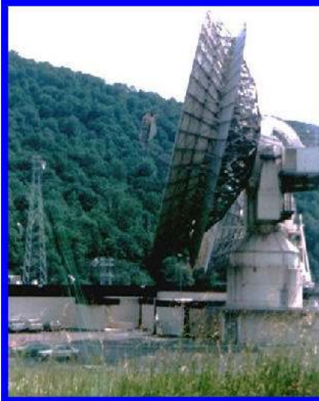
Satellite ground terminal at Etam, West Virginia, connecting Europe and the US via Intelsat IV
