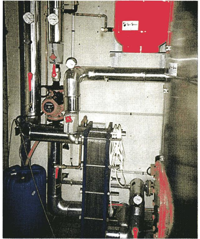
Figure 10. The technical premises in Castres Hospital showing the heat exchanger, expansion chamber and part of the hot water storage tank.
