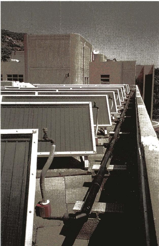
Figure 20. Part of the collector array on the roof of Bastia Hospital
