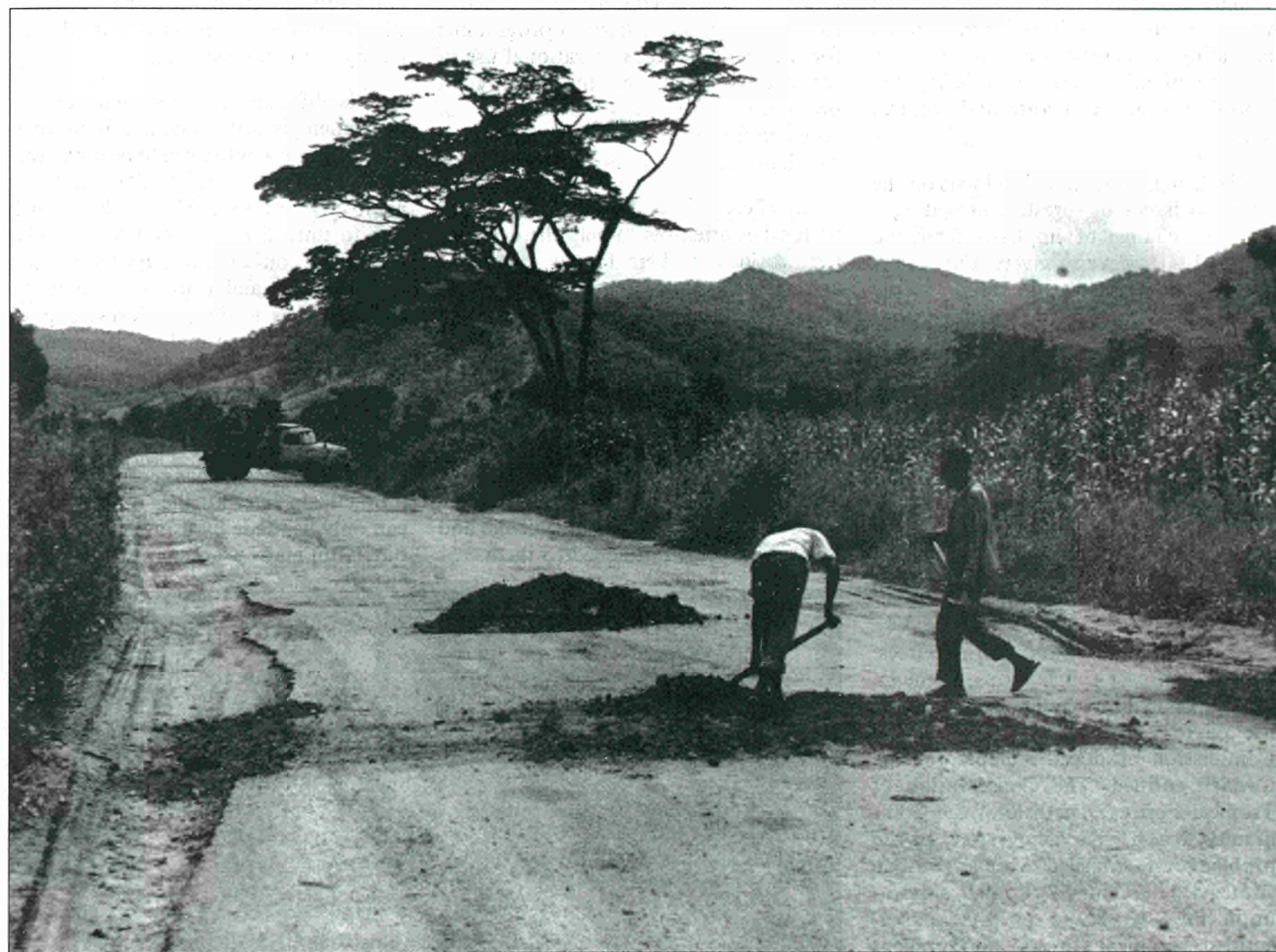
Tanzania — dealing with the potholes before they become craters
