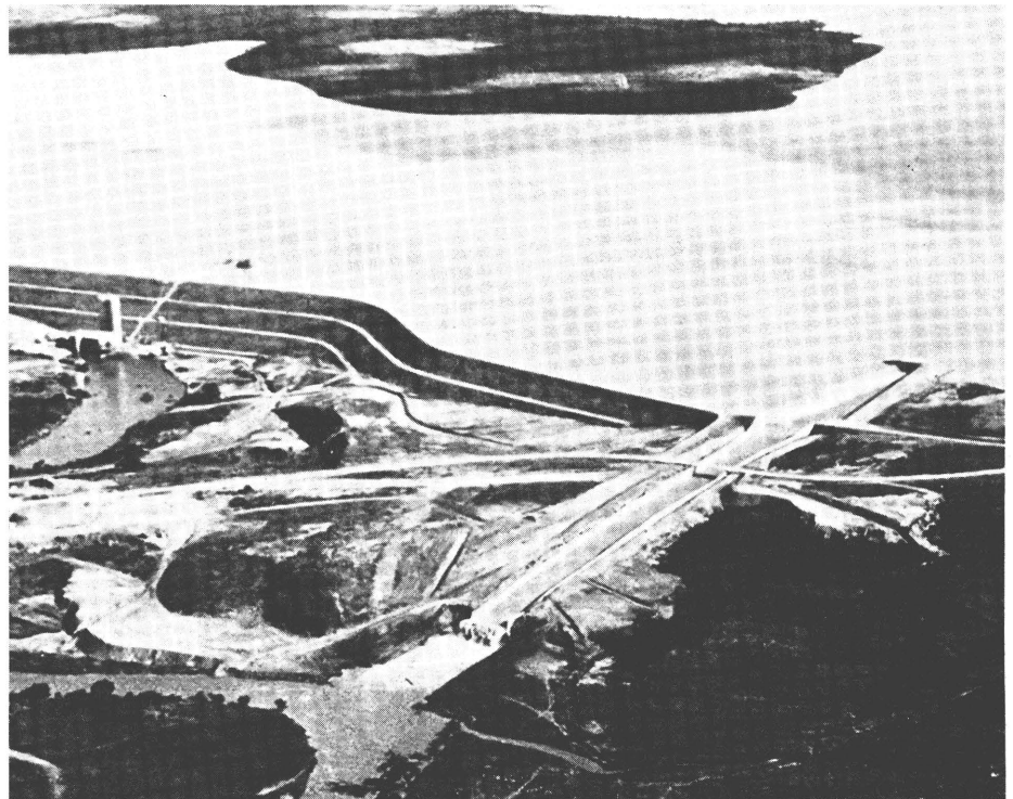
A view of the dam showing the spillway (right) in operation
