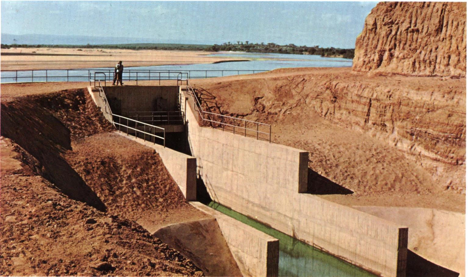
bank of the river, thanks to the construction of a water intake, an irrigation canal and the corresponding infrastructure.
